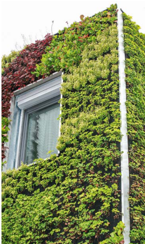
Green roof and green façade of the Weiz town hall in Styria (Austria) © Dominika Wohlmuth
